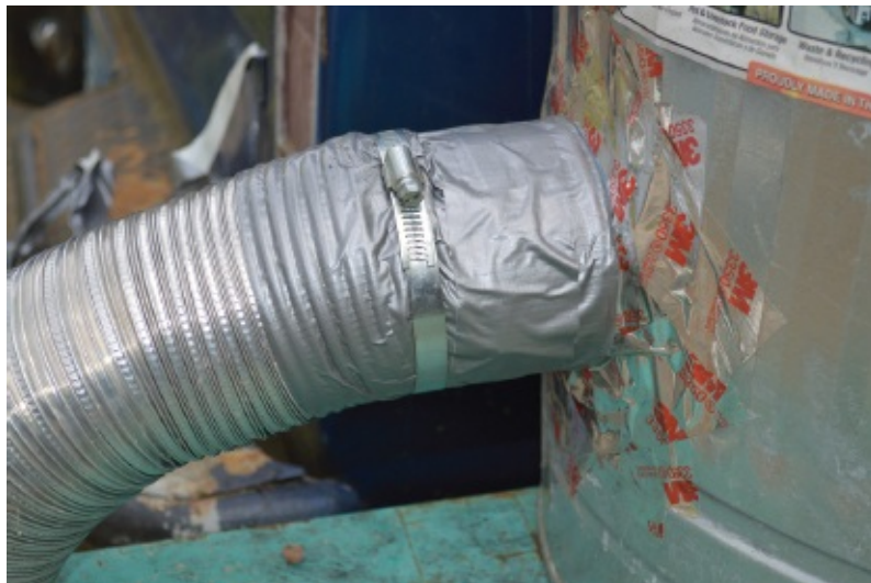
Figure 27.3 Metal hose is attached to starter.
